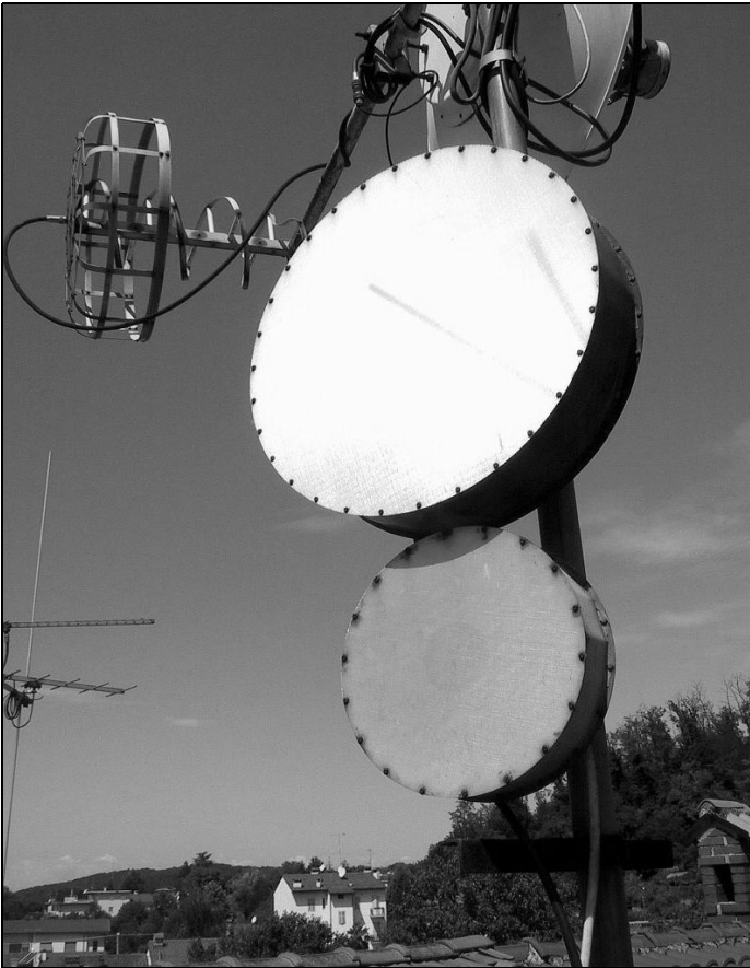
Fig 43: 23cm and 13cm SBFAs used for 1.2Mbps packet radio access.
